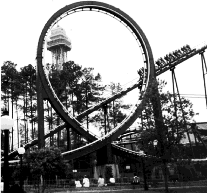
“Klothoid” shaped loop from the Shock Wave at Paramount’s Kings Dominion in Doswell, Virginia.
